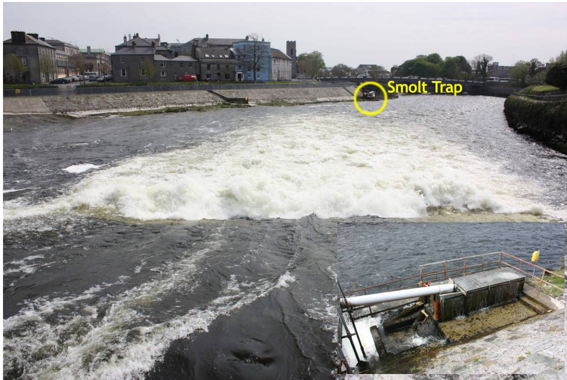
Figure 2.3.3 - Location of the Inland Fisheries Ireland smolt trap, downstream of the main weir on the River Corrib, Galway. Inset shows detail of the trap viewed from the eastern bank
